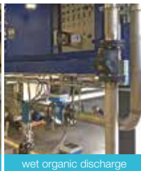
wet organic discharge
